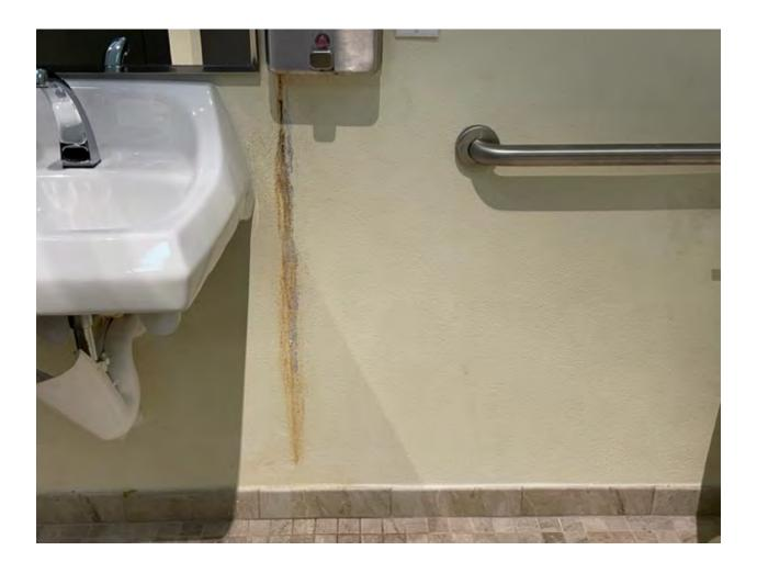
The soap dispenser in the men's bathroom is leaking & the wall needs to be cleaned & possibly repainted.
