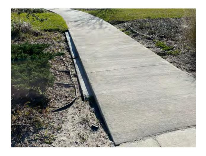
The washout on the sidewalk was repaired. We are looking into a solution to prevent the sand from leaching on the sidewalk,
